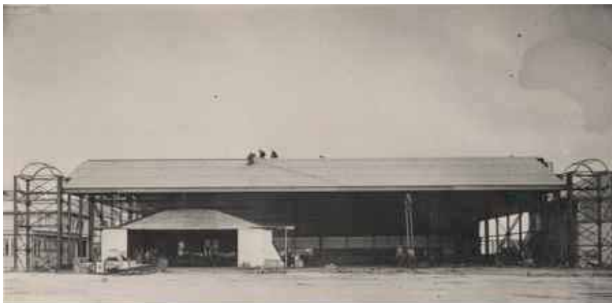
New hanger being built 1936. The original hanger is housed within the new structure.
